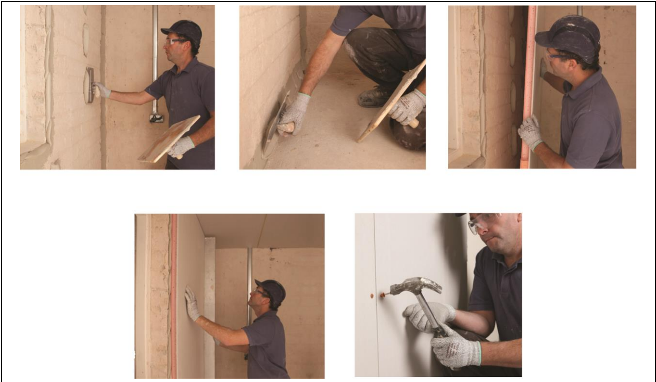
Figure 3 DriLyner TL installation details
